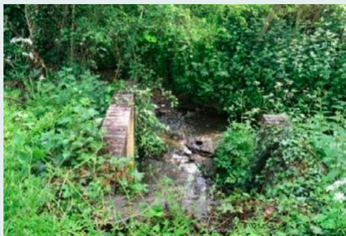
Photo: Watercourse at Stoney Stanton
