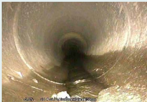
Photo: CCTV survey at Stoney Stanton
