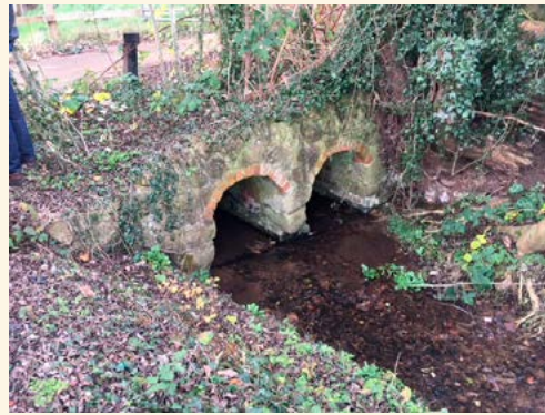
Photo: Footbridge to be removed at Breedon to increase channel capacity.
