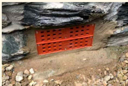
Photo: Automatically closing airbrick, Swithland
